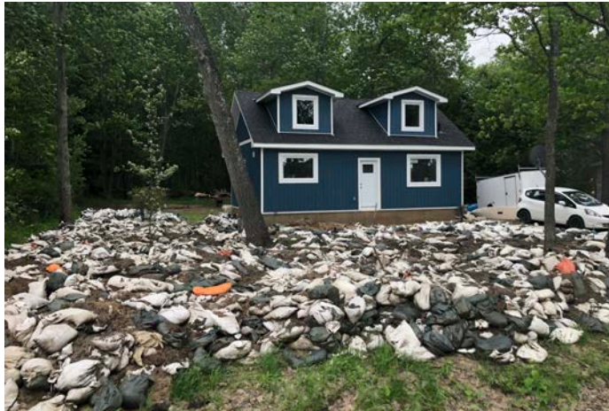
A property in Constance Bay, ON is surrounded by sandbags to protect it from the flooded banks of the Ottawa River (Cottar, 2019).
